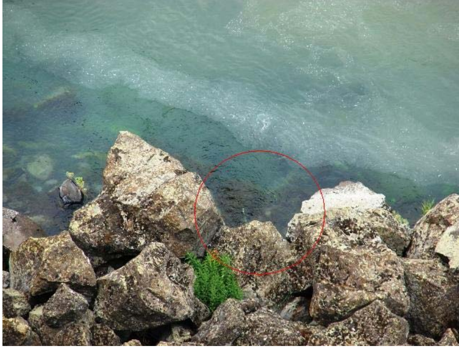
Figure 11. Closer view of MG-7 showing the high flow out into the river.
